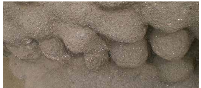
Figure 23: Injection curtain exposed [8]
