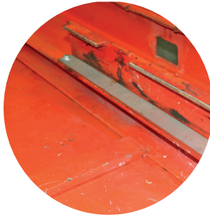
② Lower running rail inside the platform, running rail with wear strip on the running surface
